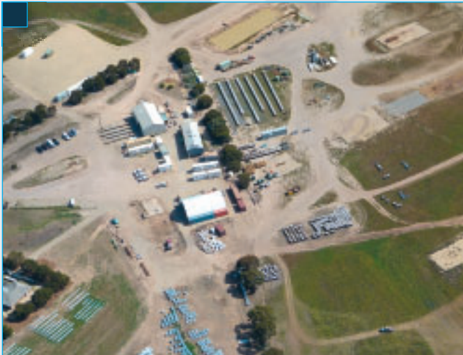
A busy worksite processing core at Hillside.
